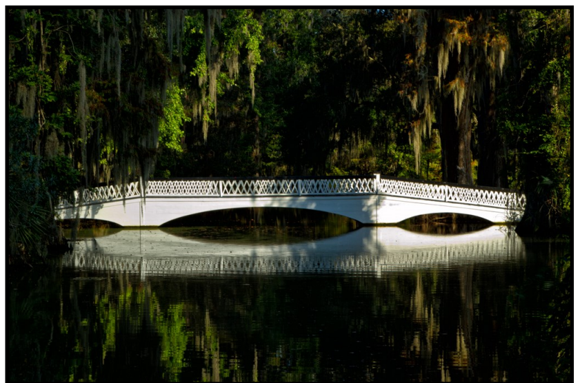
Footbridge, Charleston, South Carolina by Loye Stone
